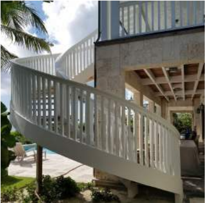
Stair cases & Railings
